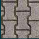
INTERNAL ROADS INTERLOCKING BLOCKS/ TREMIX CONCRETE ROAD
