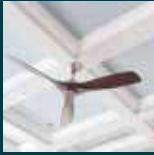
CEILING ACRYLIC EMULSION PAINT/ OIL BOUND DISTEMPER
