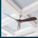
CEILING ACRYLIC EMULSION PAINT/ OIL BOUND DISTEMPER
