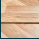
FLOOR LAMINATED WOODEN FLOOR
